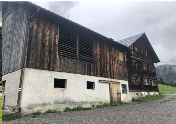
Figure 7. House Nigsch view from front Photograph: Energy Institute Vorarlberg
