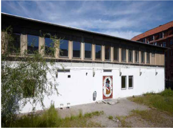
Figure 5. Façade facing garden before renovation
