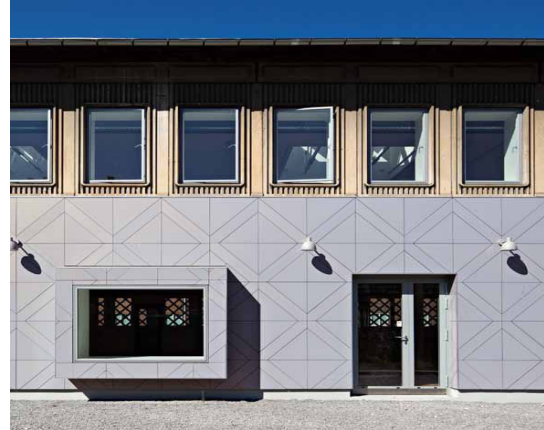
Figure 6. Façade facing garden after renovation
