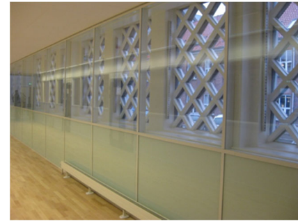
Figure 4. Façade facing inside after renovation
