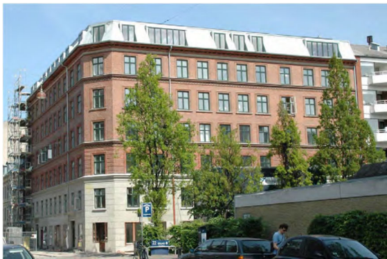
Figure 1. Façade of Ryesgade 30 after renovation including new roof and penthouse apartments. Ground floor has commercial premises.
