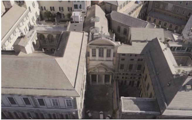
Figure 1 The former University Library, in the space of the Jesuit's Collegium Church (in the middle, XVII C.). Actually abandoned, it is under analysis by the School for a complete renovation, restoration and reuse.
