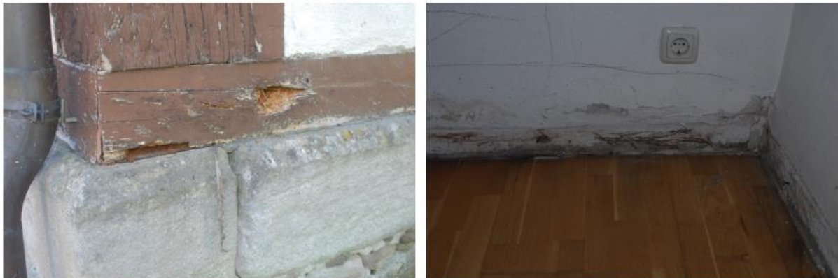
Figure 1. (a) significant loss of the wood cross-section, (b) remains of the fungus can still be seen
