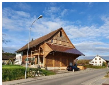
Figure 6. Rural building, Seegräben CH
