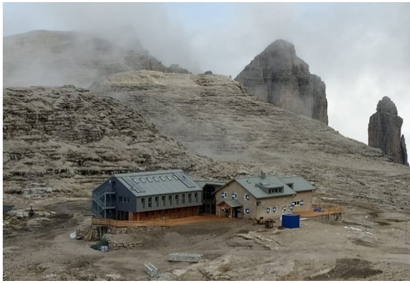
Figure 1. Picture of “Rifugio Boè”. The building consists of two parts: the new extension (left) and the renovated existing part (right) ©Giovanni Inama, Fanti Legnami S.r.l.
