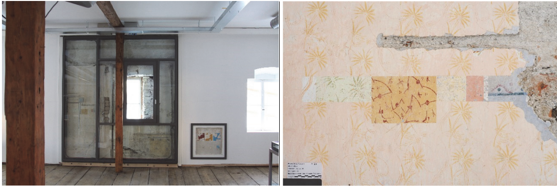
Figure 2. Reversible internal wall insulation on the upper floor of the Alte Schöfflerei. The insulation glass in front of the wall presents evidence from earlier use phases of the building (right picture). Next to it on the right Aerogel plaster was applied as internal wall insulation with a reversible mortar to protect the original surface.
