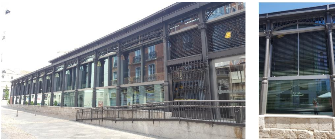
Figure 5: Multifunctional façade installed in Mercado del Val (Source: Own source)
