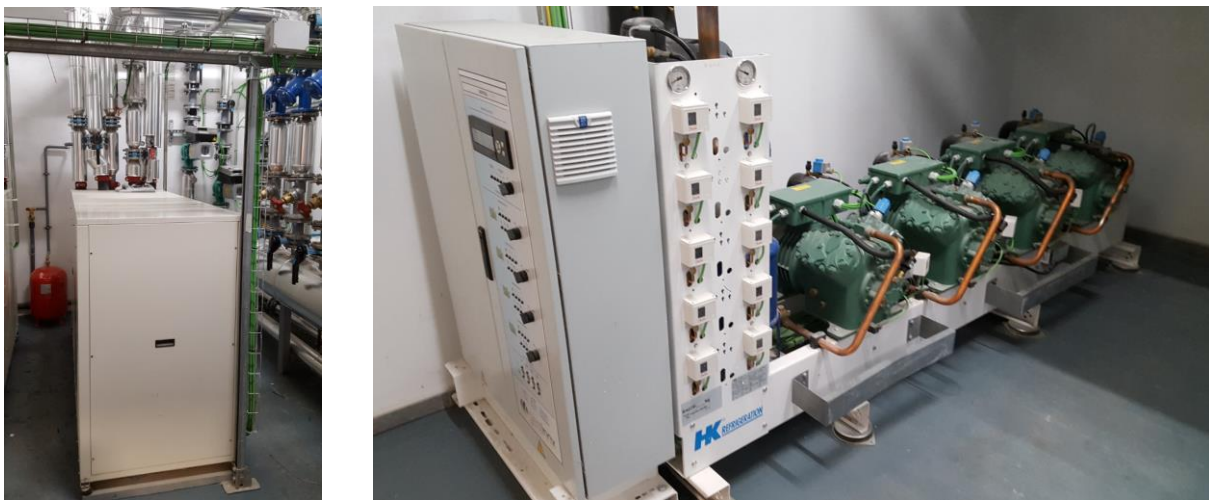
Figure 6: Reversible geothermal heat pump (left) and centralized fridge system (right) (Source: Own source)
