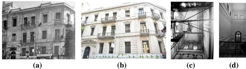
Figure 2. (a) Main façade before interventions, (b) main façade after interventions, (c) staircase before interventions, (d) staircase after interventions (first author's Ph.D. research)
