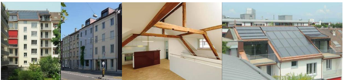
Figure 6. MFH building Feldbergstrasse (BS-CH). Source: Viridén + Partner AG. Photo: © N. Mann.
