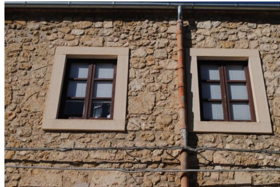
Figure 2. West-oriented façade with mp2.
