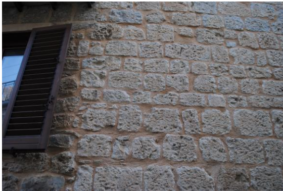
Figure 1. South-oriented façade with mp1.
