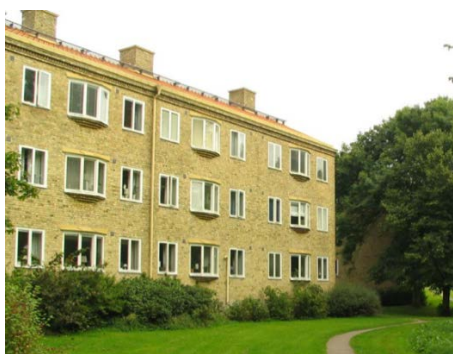
Figure 5. Company B, area from the 1940s, before renovation. Photo: Company B
