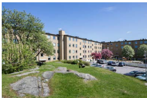
Figure 1. A residential area with replaced brick facing the courtyard and new board material on the more exposed outside facades. Photo: Private company
