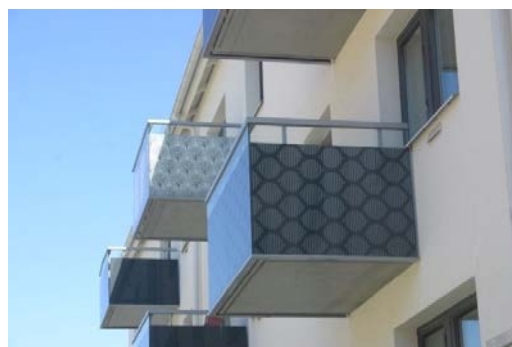
Figure 4. Company A, a 1950s area where façade, balconies and windows have been altered in a recent renovation. Photo: L. Thuvander
