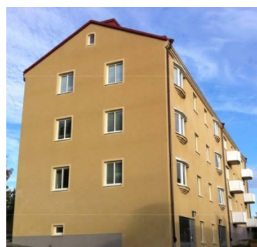
Figure 6. Company B, building in same area as Fig. 5 after external insulation, new plaster and windows. Photo: L. Thuvander
