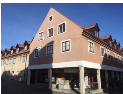
Figure 7. Company C, the 1973 property after replacement of windows. Photo: M. Legnér
