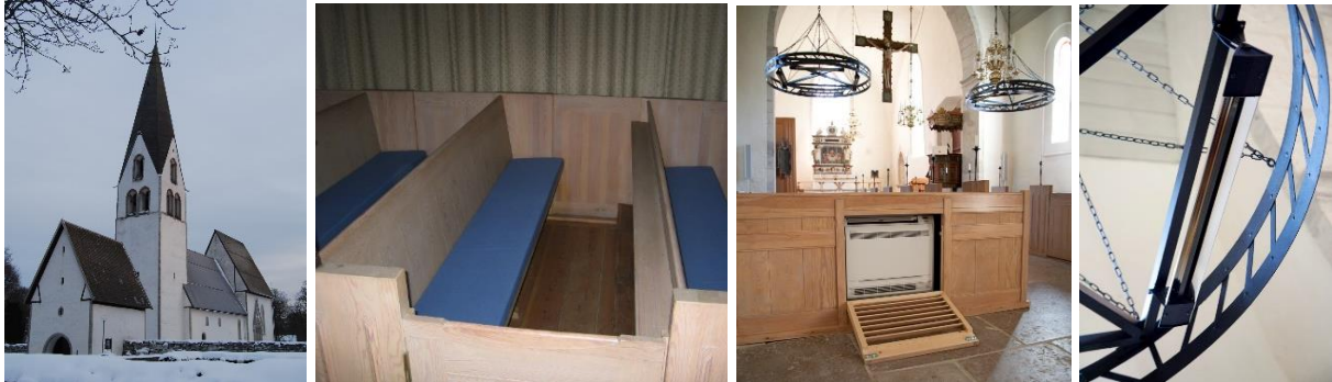
Figure 2: a) Garda church, b) the church benches with integrated heating foils in the back and radiators below the seat, c) the heat pump and overhead radiators) detail of overhead radiator
