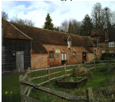
Figure 1. External view of the education centre.
