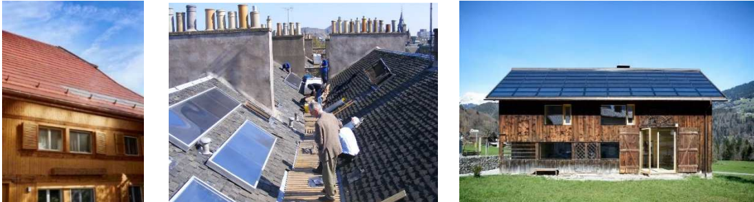
Figure 4: left: colour modules terracotta of PV © Solaragentur Prix Solaire Suisse 2018, Maison rurale Galley, 1730 Ecuwillens/FR; middle: solar thermal units on ten protected blocks of flats in the City of Edinburgh. © HES; right: side view of the House Breuer (Austria) with non-reflecting PV modules with a dark background ©FG Marcello Girardelli
